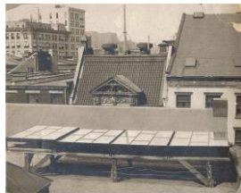
Fig. 1 – Photo with the first solar panels installed on a New York City rooftop in 1884 [2].
