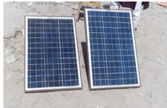
Fig. 2 – Solar panels at different tilt angles on the site.
