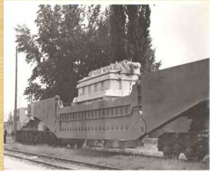
100 t furnace trafo 50 MVA ready for transportation to COS Targoviste-1978
