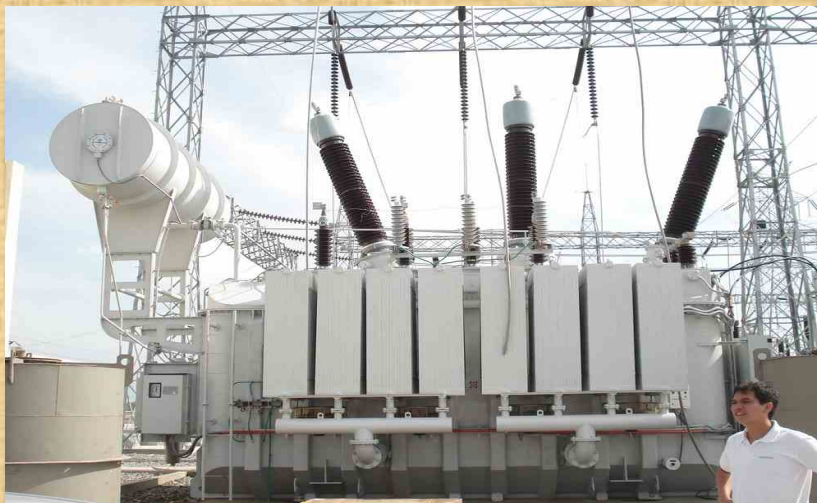
Interconnection Auto trafo 150 MVA 220/110 kV for Philippines
