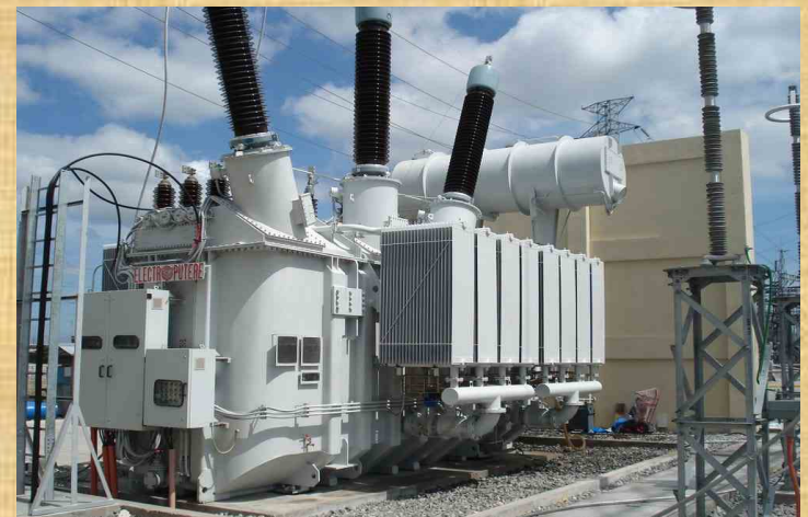
Interconnection Auto trafo 150 MVA 220/110 kV for Philippines
